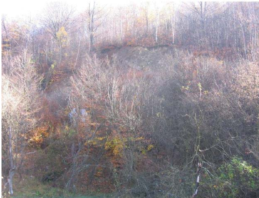
Fig. 5. Breaking phenomenon caused by sinking of the land on the slope from eastern part of the heap
